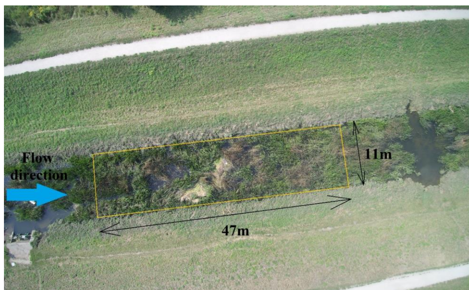
Fig. 2. The study site of the bird's-eye view photo (yellow colour indicates the exact contours of the modelled section of the Ślęza River bed)
